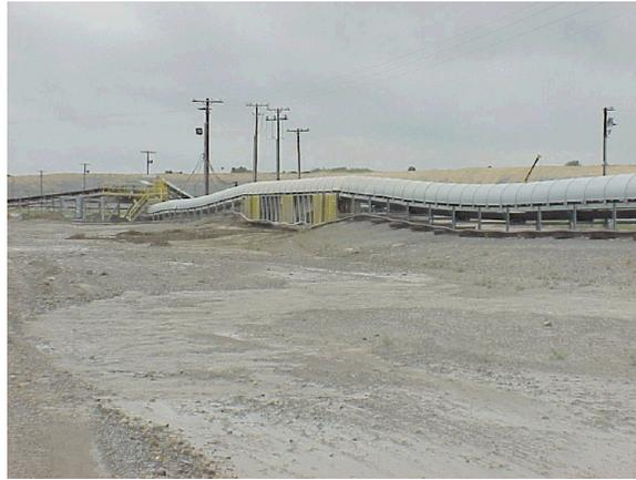
**Figure 4.29:** Covered conveyor belt for limestone transport (Copyright Halliburton Energy Services).
