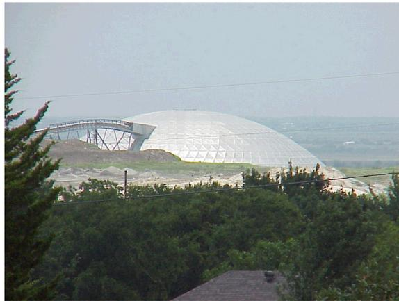
**Figure 4.30:** Exterior view of dome storage unit with conveyor loading port (Copyright Halliburton Energy Services).
